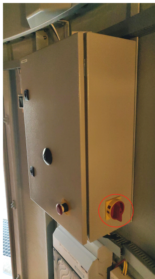
Fig. 1: Dome control box - red: main switch
