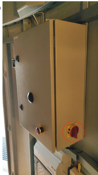
Fig. 1: Dome control box - red: main switch
