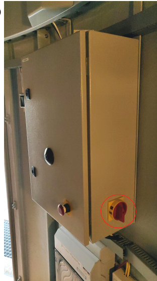
Fig. 1: Dome control box - red: main switch
