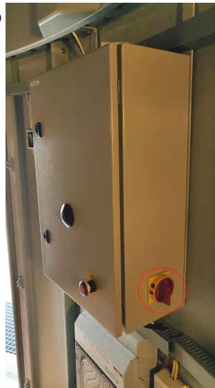
Fig. 1: Dome control box - red: main switch
