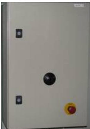
Control box with the emergency button
